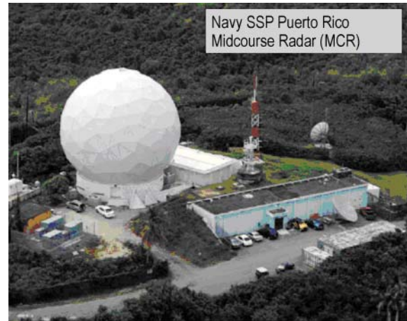
Wideband, Coherent C-Band Radar 3MW peak transmit power 0.5 M range resolution @ 500 Mhz WB LFM 15.24 M dish diameter
